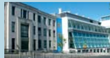
The Dainton Building, which houses the Department of Chemistry, has been extensively refurbished
