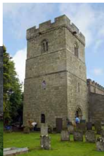
Bradbourne church - tower
